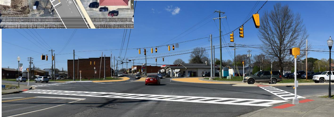
Project Int-05 conceptual rendering from person-level perspective showing the improved intersection lighting, curb bulb-outs and high visibility marked crosswalks.
